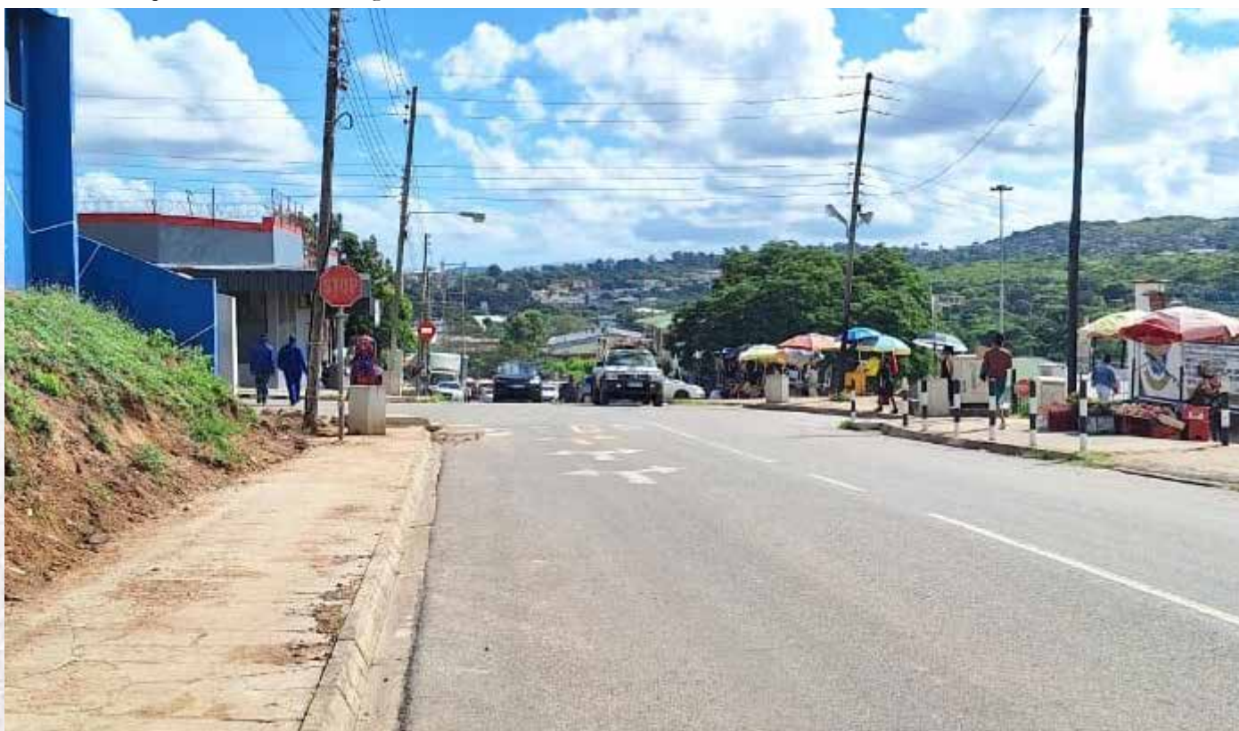
Figure 4.1 Showing City Surfaced Road Infrastructure- Mahleka Street
