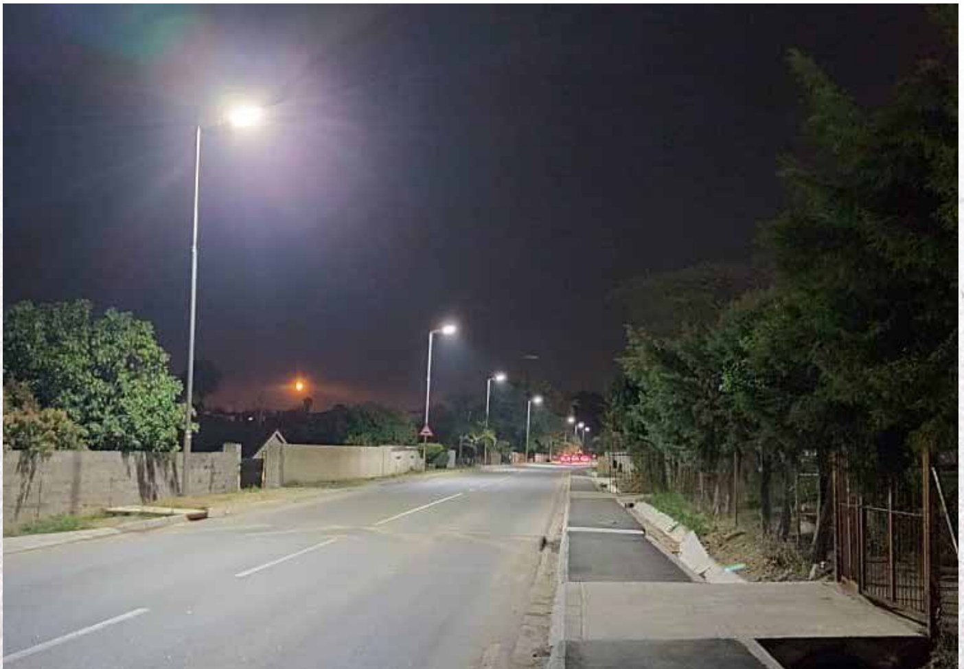
Figure 4.2 Showing Solar Illuminated Street Lighting
